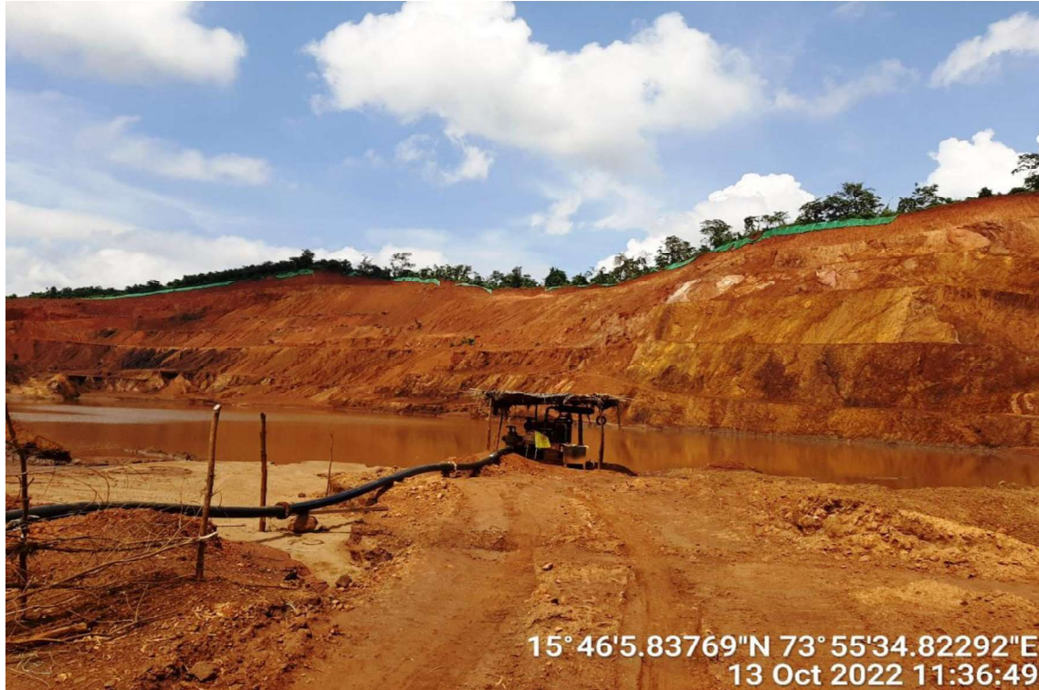
Photograph-1: Portion of working bench of mine, collapsed due to rain.
