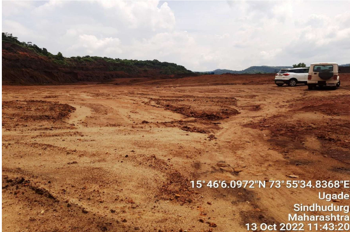
Photograph-3: Earlier mine pit, scrapped and leveled with overburden.
